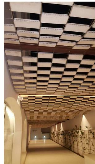
***Technical details.*** Square meters installed: 353 - Number of sheets: 161 - Size of the ceramic tile: 25 x 10 x 3 cm - Fretwork: 50% - Material of ceramic tiles: terracotta of 2 colors - Mesh and support for façade: AISI 316 stainless steel - Mean length of sheets: 2.37 meters - Construction time: 15 days - Architecture firm: MIXI Arquitectos.
